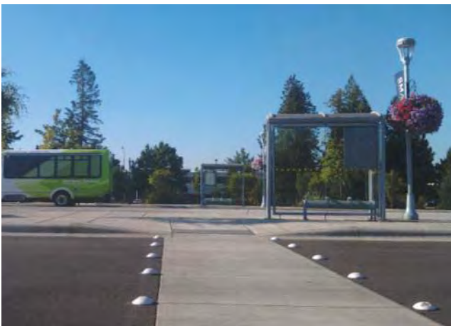
Curb ramps with gradual slopes and large transit pads at the SMART Central transit center can accommodate users in wheel chairs or with other special needs.
