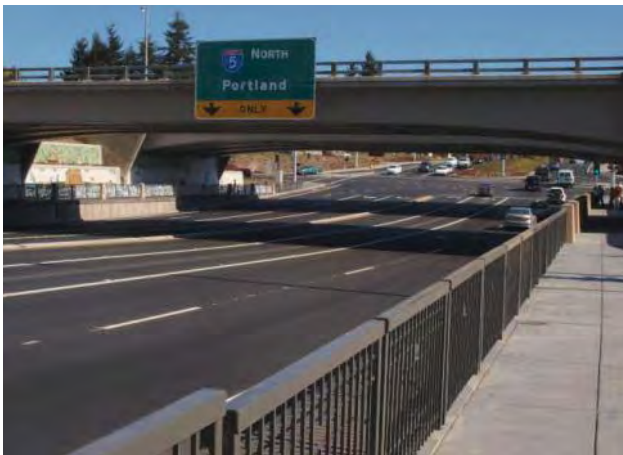
Looking east to the I-5/Wilsonville Road interchange. Interchange areas have the most restrictive access spacing standards to ensure safety and mobility.
