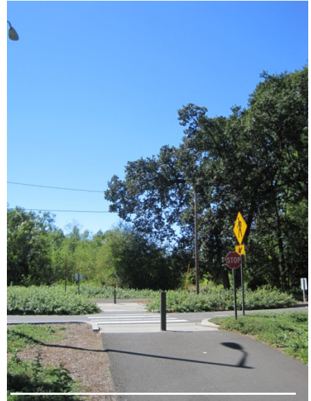
Enhanced Pedestrian and Bicycle Crossing Example
