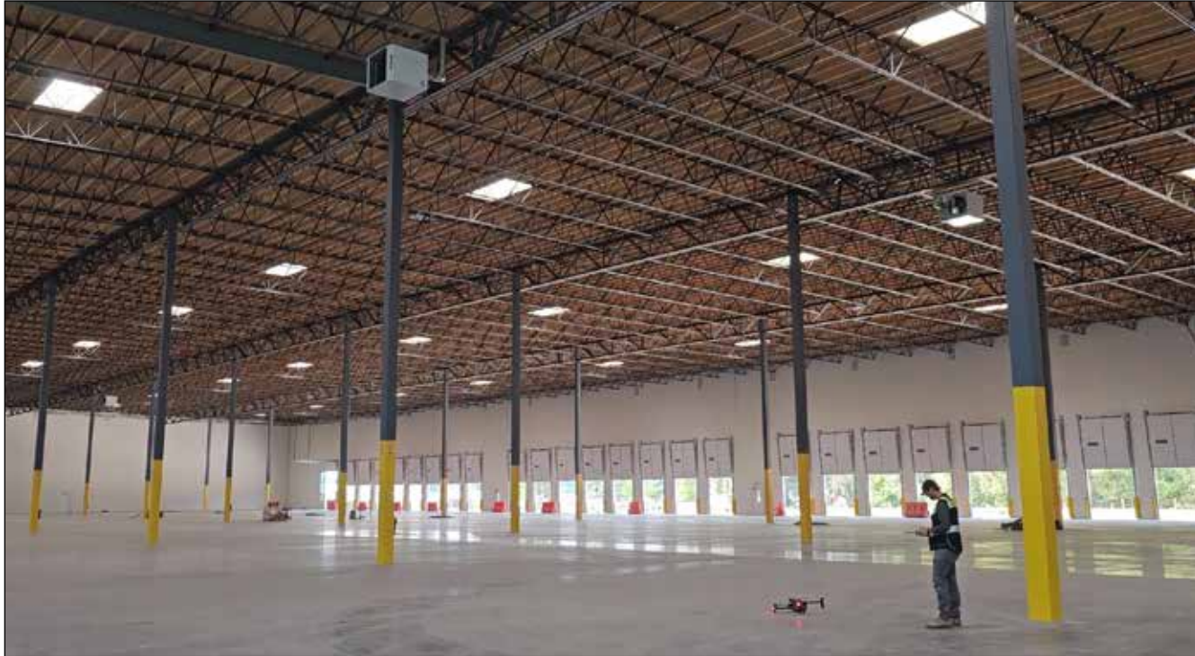
City building Inspector Carl Brown readies a drone camera to ascend within the interior of the Black Creek III warehouse in the Coffee Creek Industrial Area. Drone technology is revolutionizing building inspections by allowing safer inspection of areas that would historically require inspectors to climb scaffolding or ride a scissor lift.
