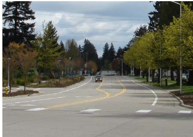
Example of a Collector - Barber Street looking east near SMART Central at Wilsonville Station transit center
