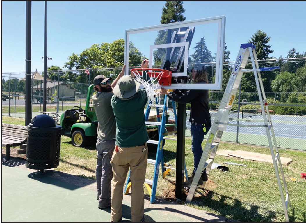
Park Maintenance staff replacing a basketball hoop.
