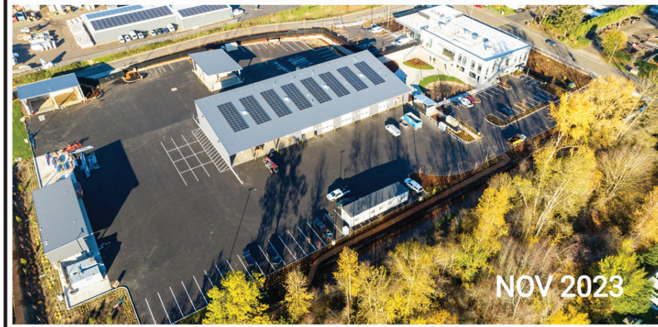
Public Works Complex (CIP #8113).
