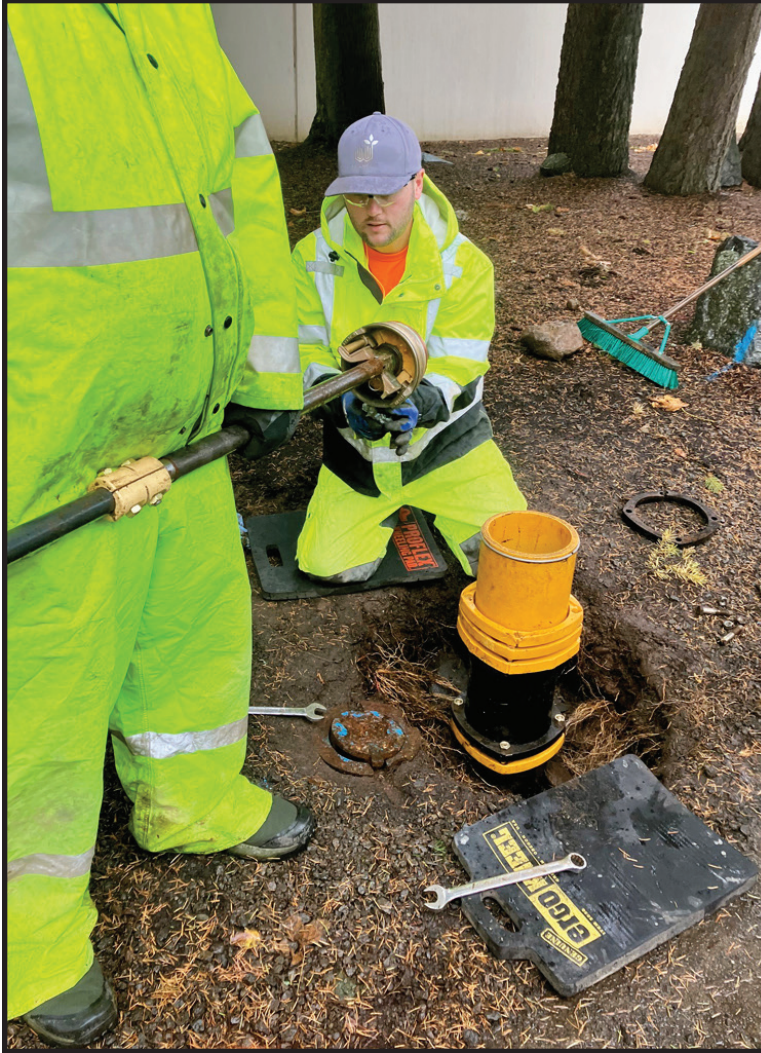
Water Distribution Technicians rebuilding a fire hydrant.
