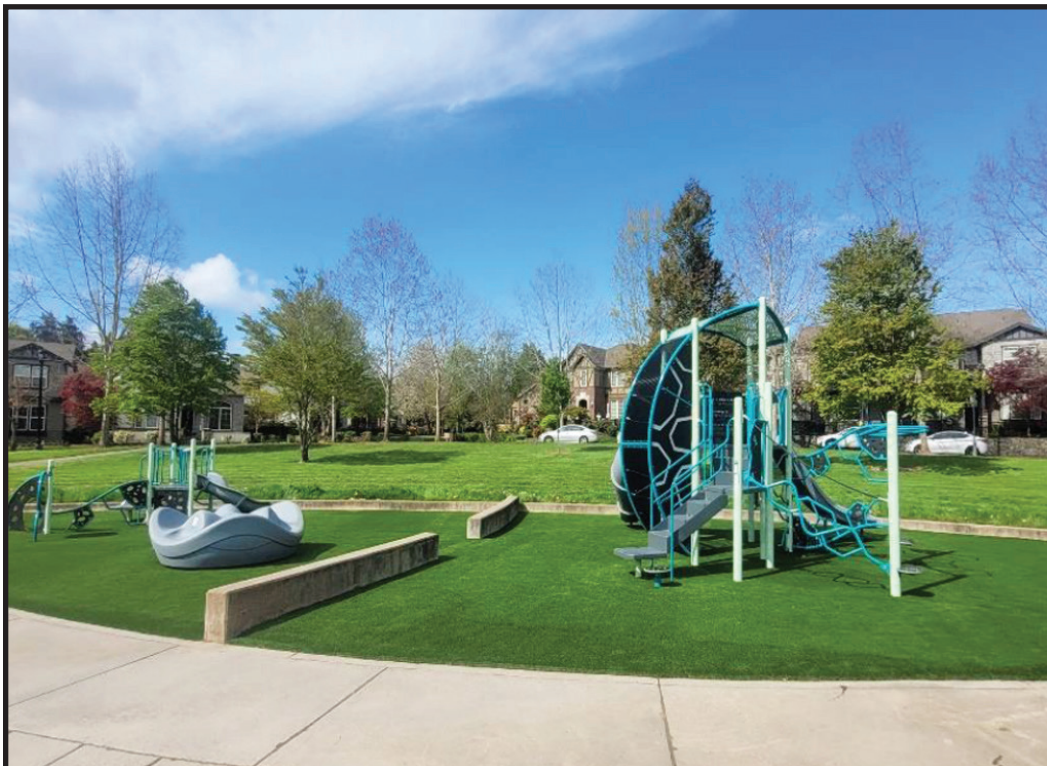
Installation of a new playground equipment at Sofia Park in Villebois (CIP #9152).
