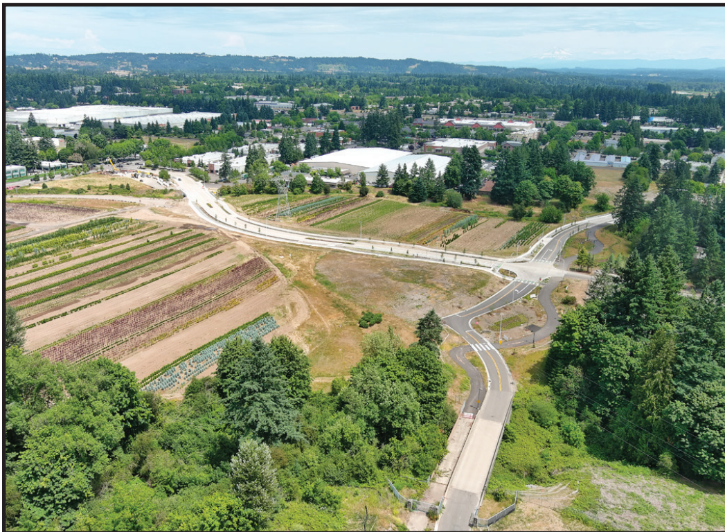
Aerial view looking northeast of a completed 5th Street/Kinsman Road Extension (CIP #4196).
