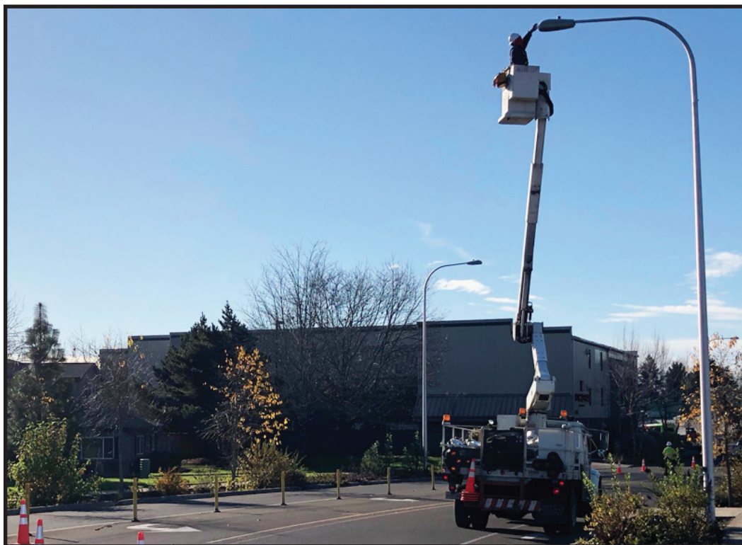
LED streetlight conversion project - light installation.
