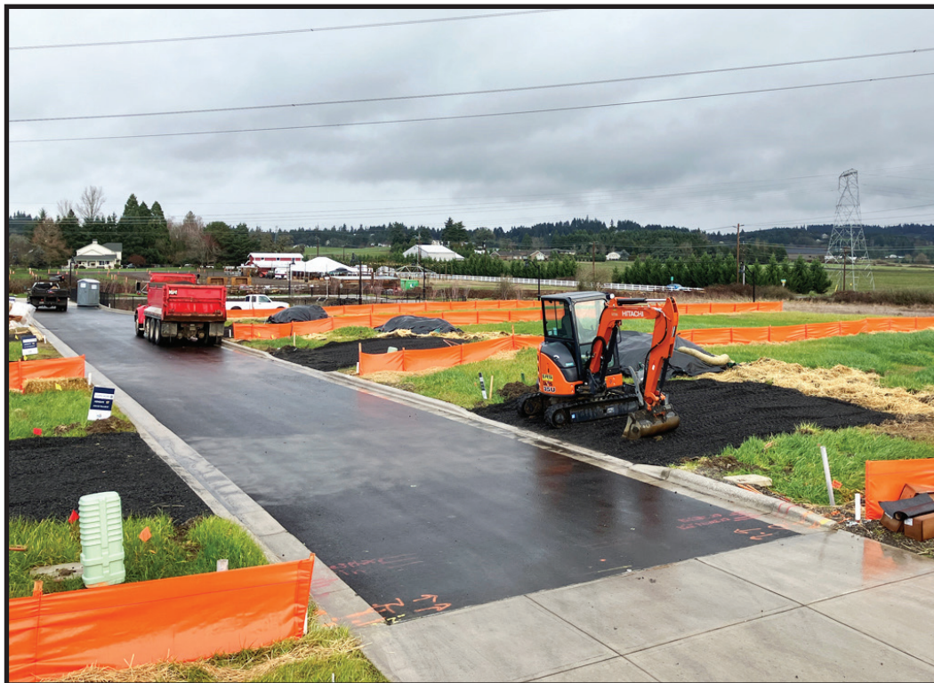
Frog Pond West erosion control.
