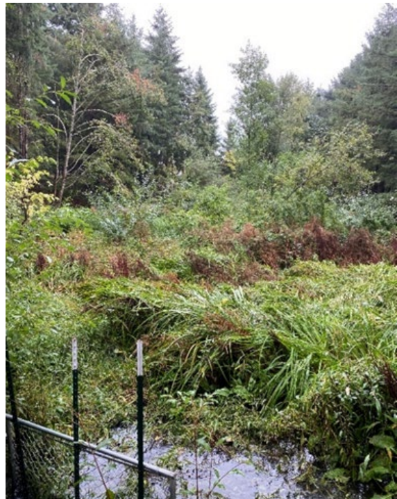
Dense, overgrown vegetation and accumulated sediment, combined with a lack of an outlet control structure, limits Library Pond's capacity and water quality function.
